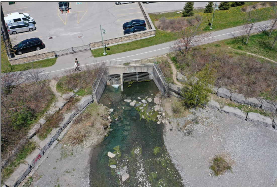
Figure 24. Stormwater outfall located near the Ajax Water Supply Plant. Source: TRCA, 2021.
