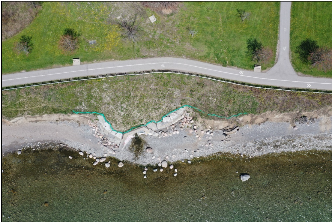
Figure 7. Aerial view of headwall repair conducted in 2020. Source: TRCA, 2021.
