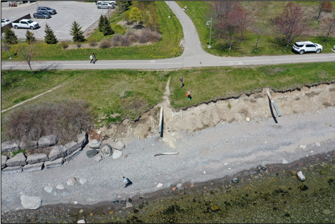
Figure 23. Infrastructure exposed along the Ajax waterfront. Source: TRCA, 2021.
