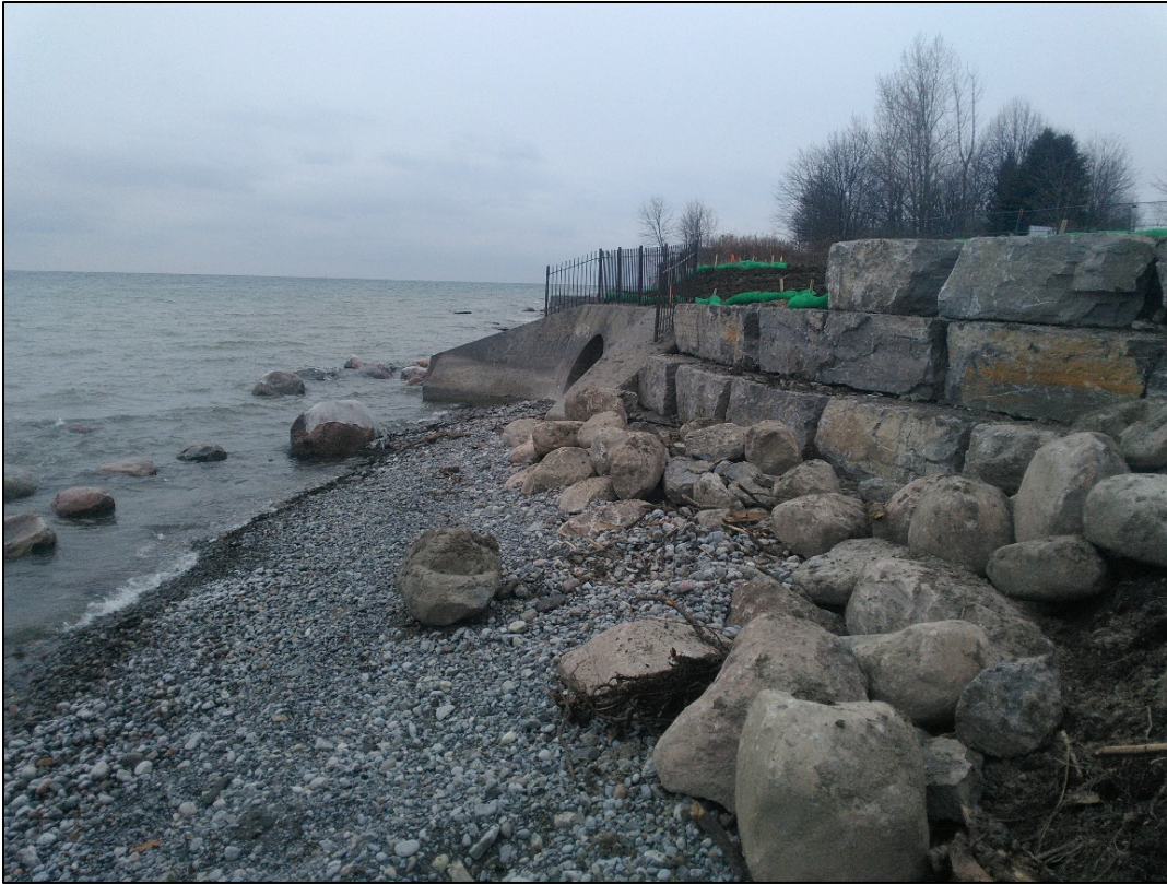
Figure 8. Shoreline view of headwall repair and armourstone structure from 2020. Source: TRCA, 2021.
